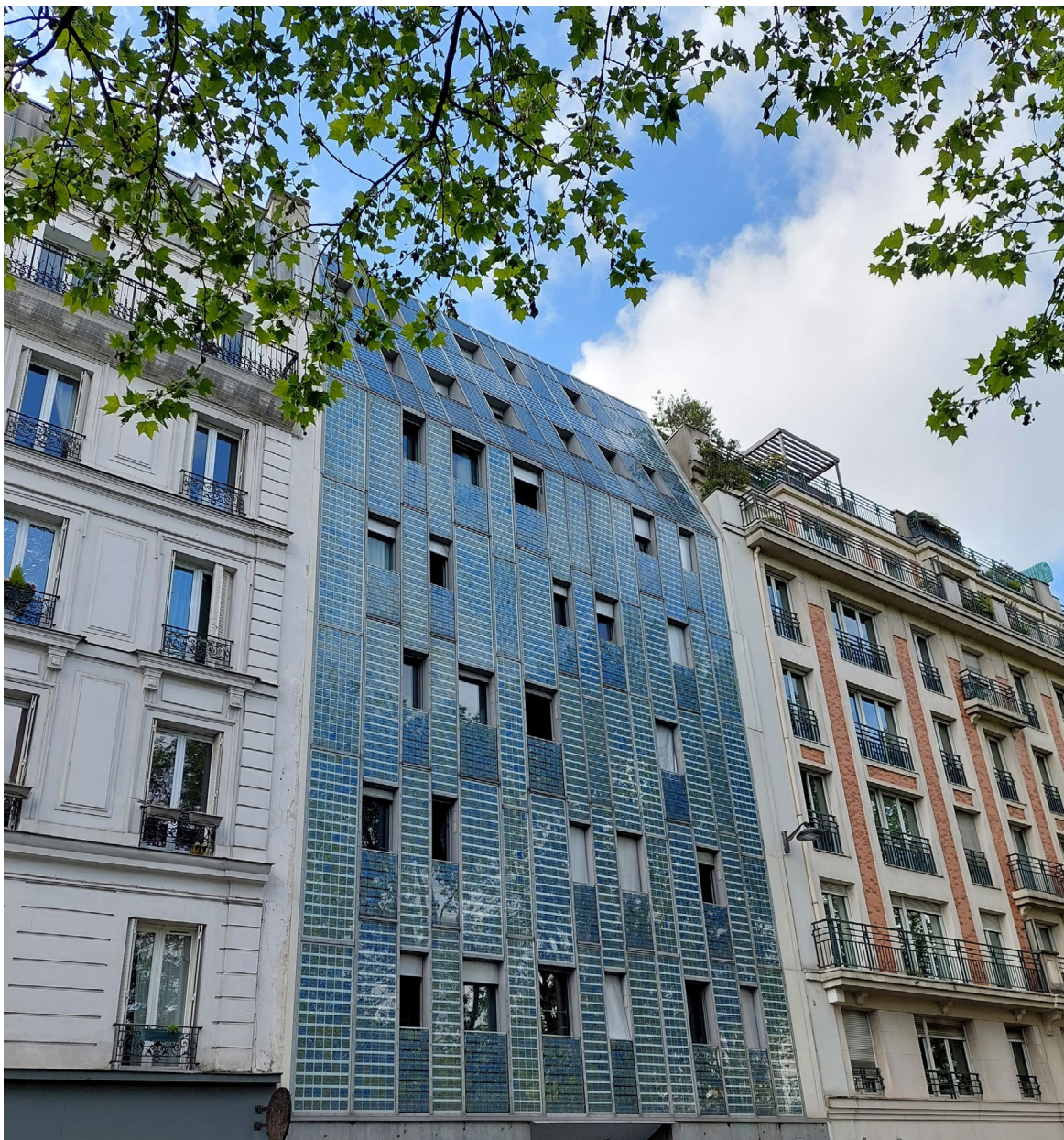
Façade photovoltaïque, Paris – E. Saadi, architecte. © Roland Peltekian
